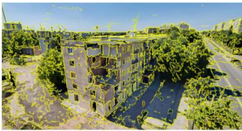
Figure 5. Output of Felzenszwalb segmentation (scale = 300, sigma = 0.9, min_size = 50) on a damaged building image. Yellow contours mark regions grouped by local color and texture similarity.
