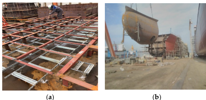
Figure 4. (a) cableways during the block stage, (b) the bigger mega block.
