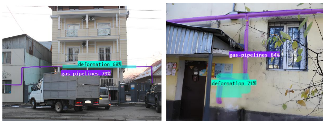
Figure 4. Example of automated detection of deformations on external gas pipelines using the trained models.
