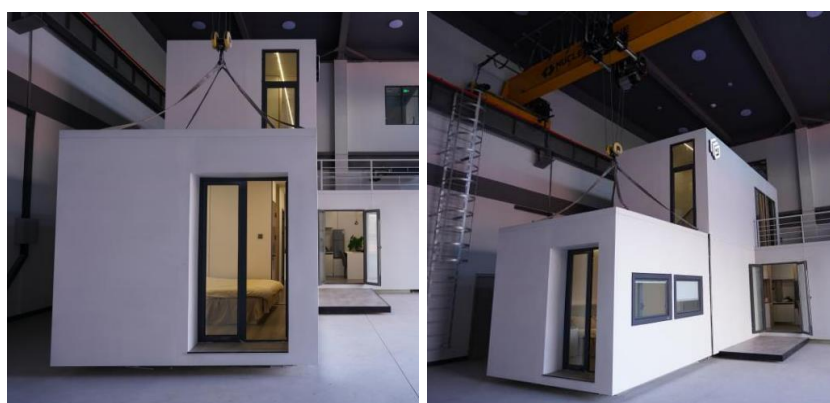
Figure 7. Module lifting diagram.
