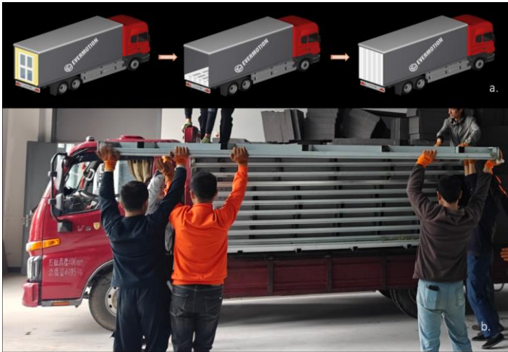
Figure 9. Module transport for Magic Box 1.0 (a. concept b. Field photo).
