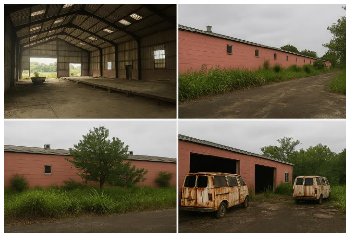
Figure 1. Defunct Benue Burnt Bricks Factory, Otukpo, Nigeria.
