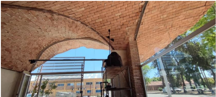
Figure 17. Real size model of the interconnection of tunnels constructed to monitor different parameters.
