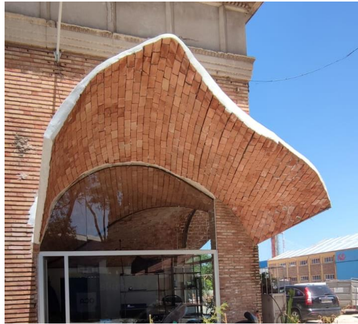
Figure 18. Experimental model of the reflective ceiling of the tunnel before coating. Seville.
