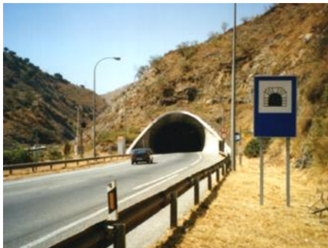
Figure 1. Black-hole effect at the entrance of road tunnel.
