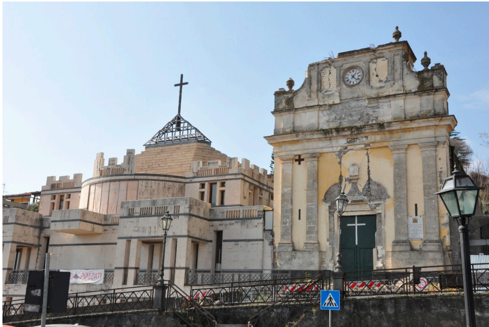
Figure 6. Parish complex of Maria SS. del Rosario in Fleri, Zafferana Etnea. On the right is the old church, renovated after the 1984 earthquake and damaged again by the 2018 earthquake. On the left is the new church, recently built with reinforced concrete anti-seismic structures, which suffered only minor damage during the 2018 earthquake. This church has always been a symbol of Fleri's identity; for this reason, it was decided to restore the entire parish complex, including the old church, through innovative structural interventions aimed at ensuring its stability in the event of future earthquakes.
