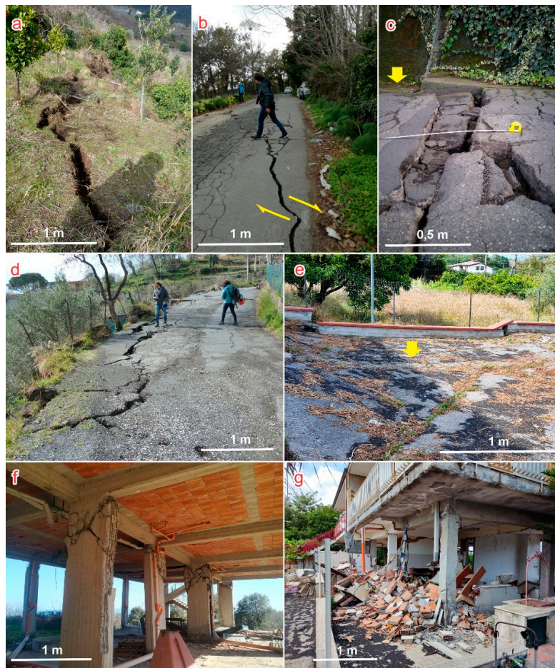
Figure 5. Effects of surface faulting on soils, roads and buildings; the yellow arrows indicate the directions of movement. (a) Extensional fractures near a slope edge. (b-c) Left transpressive fractures on road pavements. (d) Edges of seismo-induced landslide detachment. (e) Graben formed at the center of an extensional fracture system. (f) Failure of reinforced concrete of a building constructed above a fault plane. (g) Collapse of infill walls
