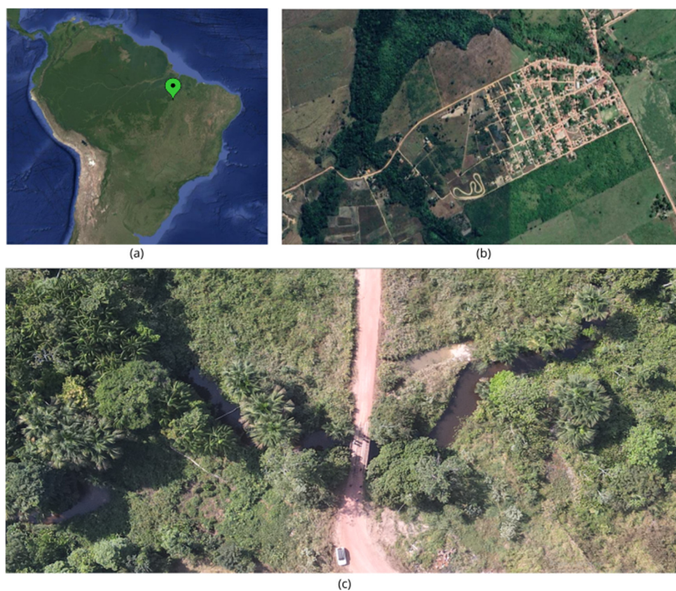
Figure 1. Location of the Janari community and the small river Água Preta: (a) Overview map of Brazil showing the location of Janari, indicated with a marker (image from Google Maps); (b) Closer view of the Janari area, as indicated in (a), showing local geographical context (image from Google Maps); (c) Aerial photograph of a small portion of the area shown in (b), taken by the research team, featuring a bridge crossing the Água Preta stream.
