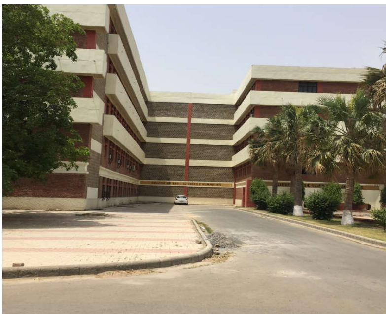
Figure 1. The multi-storey building of the College of Basic Sciences and Humanities, where A. dorsata nested on various ceiling projections (Adapted from Sihag, 2017 [22]).
