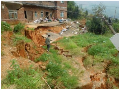
Figure 8. Downward platforms at rear of a newly failed slope.
