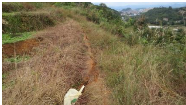
Figure 9. A tensile crack at rear edge of the slope.
