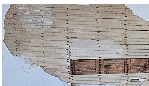
Figure 55. Batten wattle and daub - Third Island – Porto Judeu.
