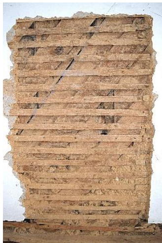
Figure 52. Double wattle and daub - Santa Comba Dão.
