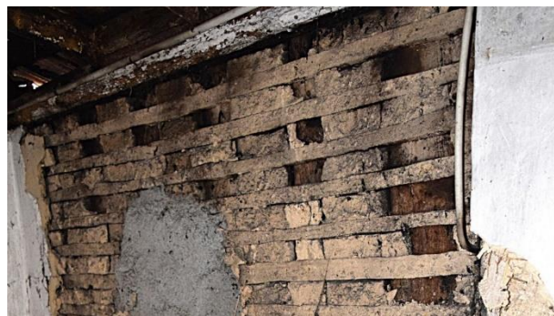
Figure 61. Insulating wattle and daub - Boassas.
