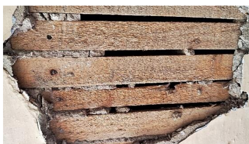
Figure 54. Batten wattle and daub - Third Island - Biscoito.
