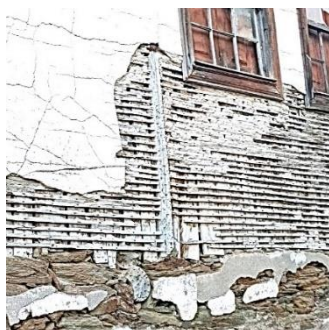
Figure 47. Simple wattle and daub - Cedovim.
