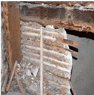
Figure 58. Wood shavings wattle and daub - Funchal.
