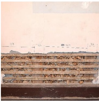
Figure 58. Wood shavings wattle and daub - Funchal.
