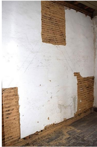
Figure 51. Double wattle and daub - Santa Comba Dão.
