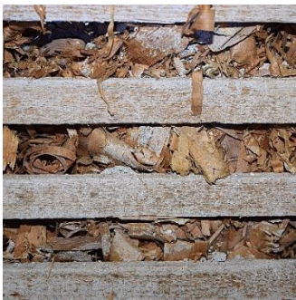
Figure 57. Wood shavings wattle and daub - Funchal.
