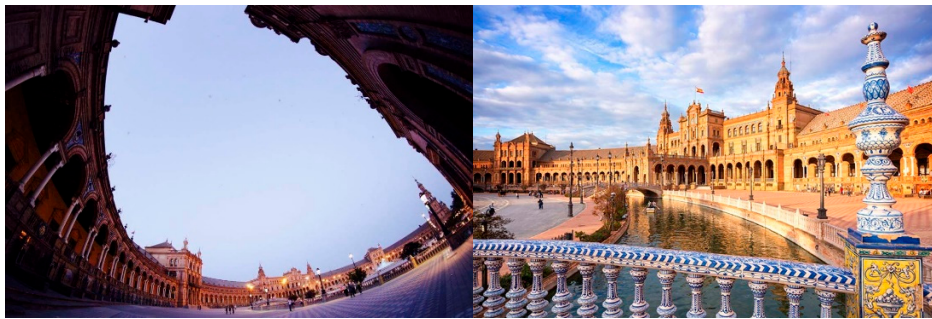
Figure 3. Plaza de Espana, Seville, today.
