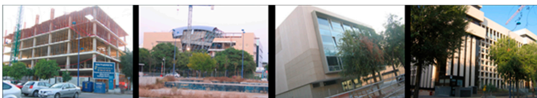
Figure 15. New construction sites in the Expo'92 area.
