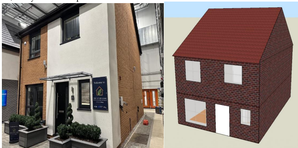
Figure 1. Front elevation of TFH in Energy House 2.0 Environmental Chamber one (left) and TFH modelled in DesignBuilder (right).
