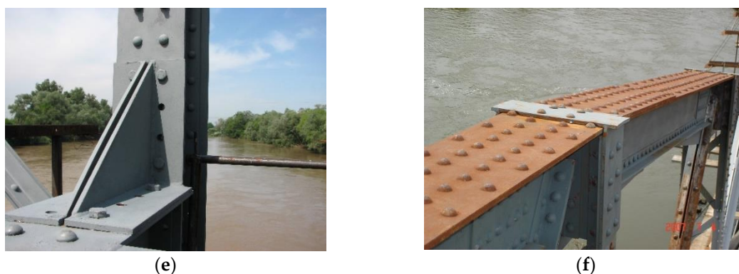
Figure 2. On-site work for bridge rehabilitation: (a) deck removal; (b) Warm post straightening; (c) sand blasting; (d) Riveting; (e) New consolidation elements; (f) Reinforcement of upper chord joint.
