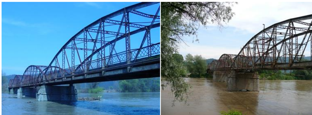
Figure 7. The general view of the Săvârșin bridge.
