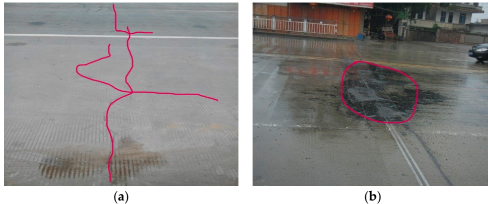
Figure 2. Observed cracks and damage in the bridge deck. a) Cracks in the link slab. b) Damage in the expansion joint.
