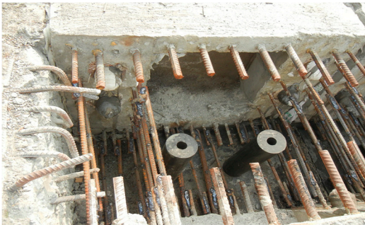
Figure 9. Photo of the continuous segment with dowels over the pier before concrete casting.
