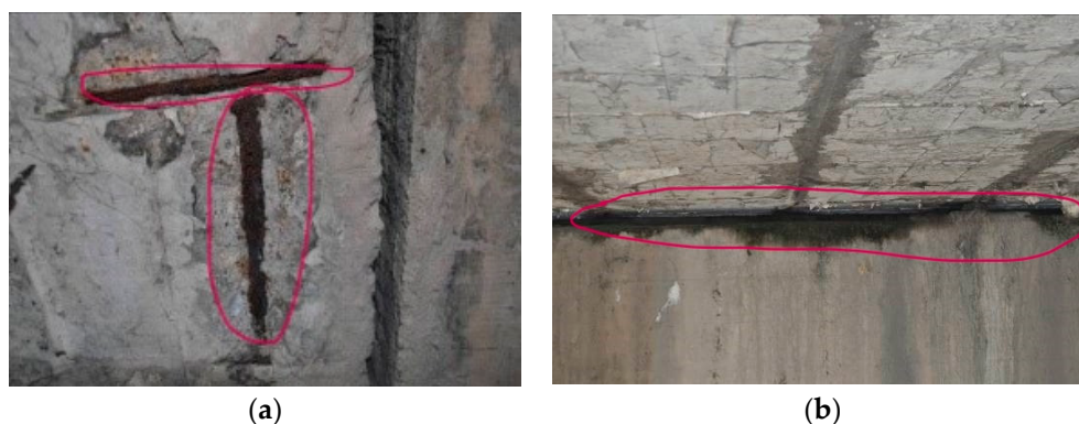
Figure 3. Views of distress in the voided slabs and water leakage on the top of the abutment. a) Reinforcement corrosion and concrete spalling at the soffit of the voided slab. b) Water leakage on top of abutment.
