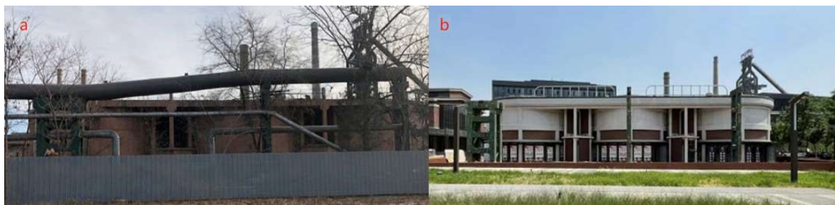
Figure 8. original building (a) by the author in 2018, case building after renovation (b) by the author in 2023.
