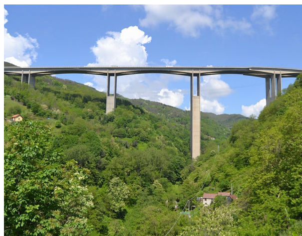
Figure 9. “Viadotto Gorsexio” with a central pillar taller than 172 m.
