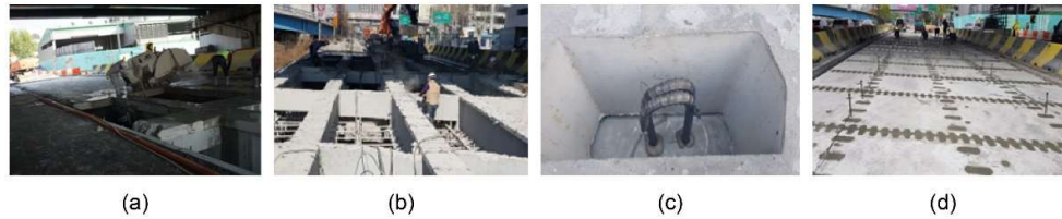
Figure 1. Case study on the removal and reconstruction of aged concrete slabs. (a) Cutting aged concrete slab; (b) Cutting rebar shear connectors; (c) Reinstallation of rebar shear connectors; (d) Complete reconstruction of new PC slab.
