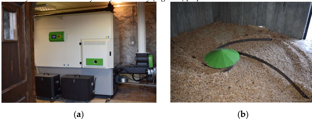
Figure 2. (a) PelleTech Biomass boiler; (b) agitator feeding system installation in Saint Vissarion Monastery, Trikala Greece [14].
