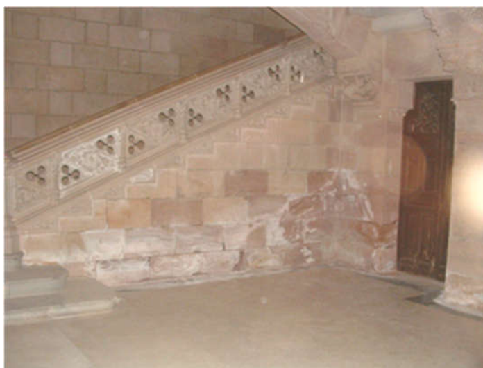
Figure 2. Efflorescence associated with rising capillary water. Seminario Mayor de Comillas (Cantabria).
