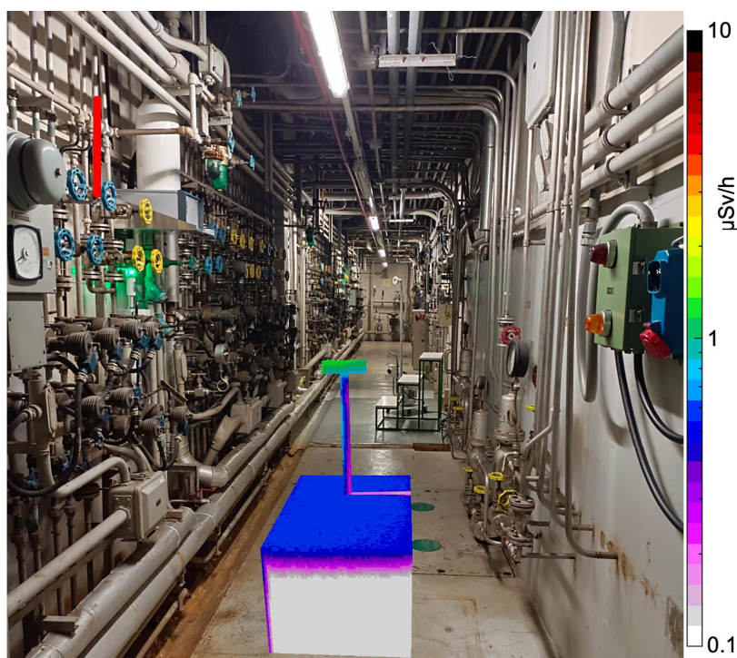
Figure 18. Simulation of a hypothetical environment to be inspected: a long tunnel with pipes, valves, cables. A 70 cm vertical pipe section, highlighted in red for clarity (top left), was assumed as contaminated with 10 MBq of ^{60}\text{Co} . The dose rate scale only refers to the UGV.
