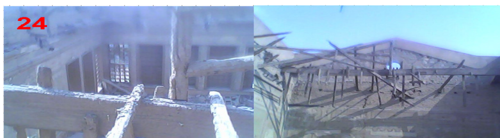
Figure 24. the truss wooden ceiling of the great throne hall after the 1972 fire.
