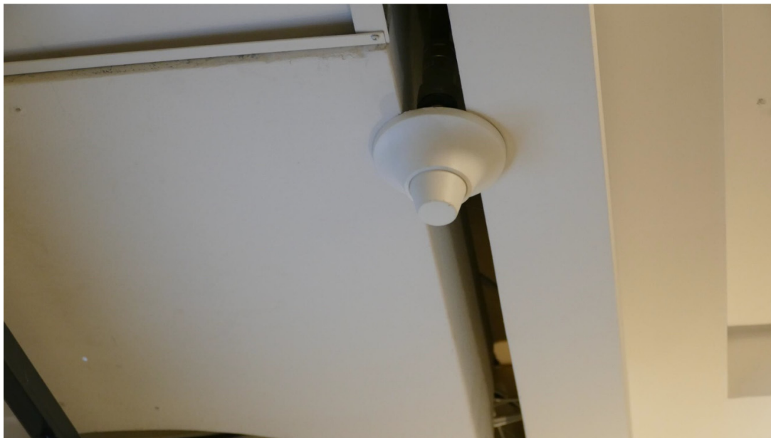
Figure 3. Microcell at Stockholm Central Railway Station, Stockholm, Sweden.
