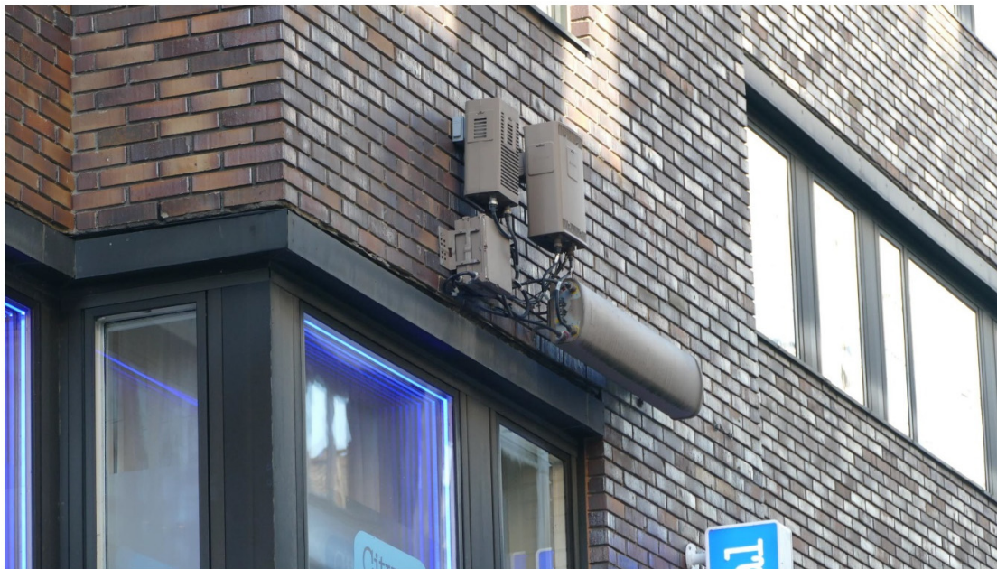
Figure 5. Low positioned base stations at Drottninggatan, Stockholm, Sweden.
