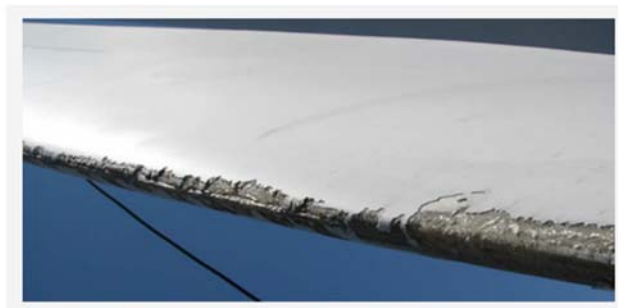
Figure 5. – Image of leading edge damage [11].
