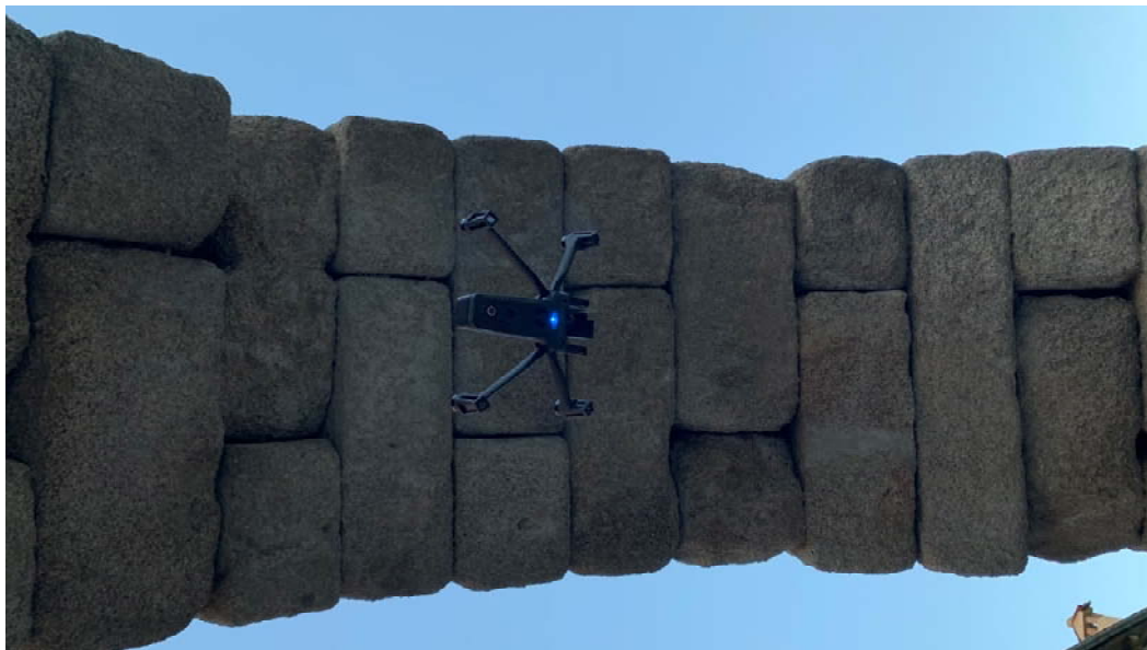
Figure 1. General view of the four-rotor drone with a thermal imaging camera used in one of the inspections, that of the Segovia Aqueduct, at a time when it was inspecting the ashlars and voussoirs that make up one of the arches, on the inside of the monument (photograph by the author).
