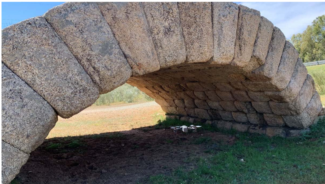
Figure 21. Quadcopter drone with thermal imaging camera used in the inspection, entering the first vault for the inspection of its intrados (photograph by the author).
