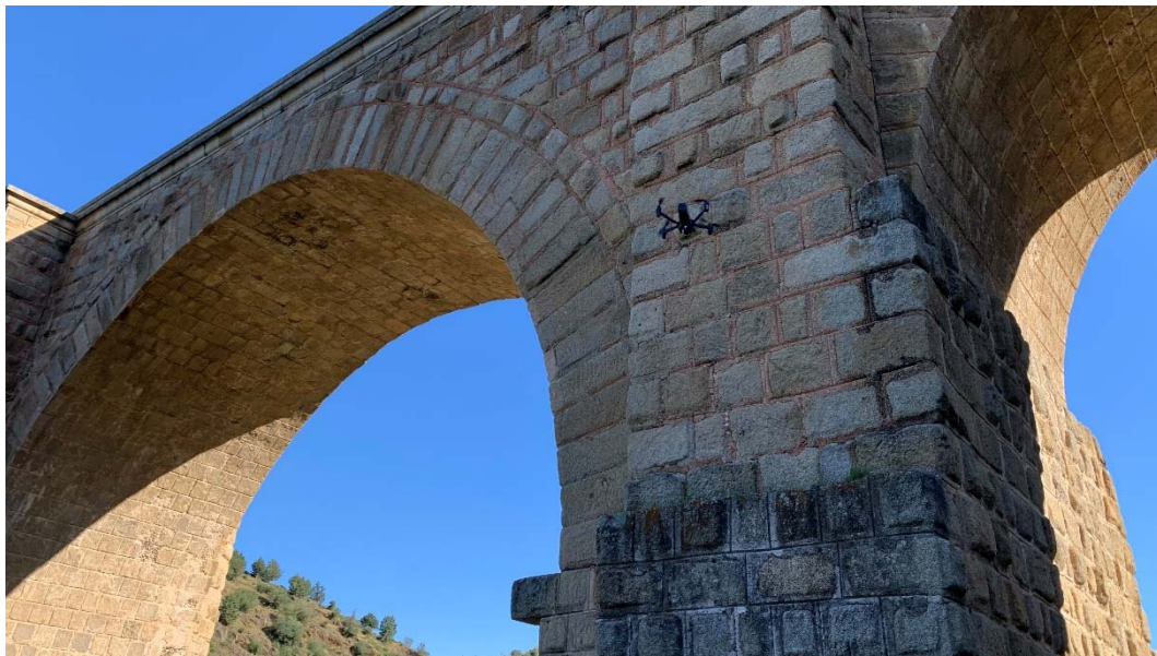
Figure 12. General view of the quadcopter drone with a thermal imaging camera used during the inspection of the first pier of the Alcántara Bridge, on its west side (photograph by the author).
