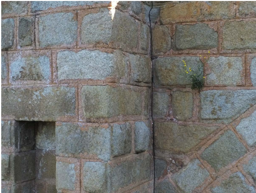
Figure 13. Photographic image captured by the drone during the flight, ascending 15 m above the position shown in Figure 12, where the lime mortar joints and the presence of organic matter and vegetation can be observed (photograph by the author).
