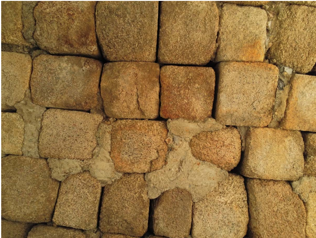
Figure 22. View of the intrados of the first lowered vault, in a photographic image taken with the drone, where altered granite elements and remains of cement mortar were found (photograph by the author).
