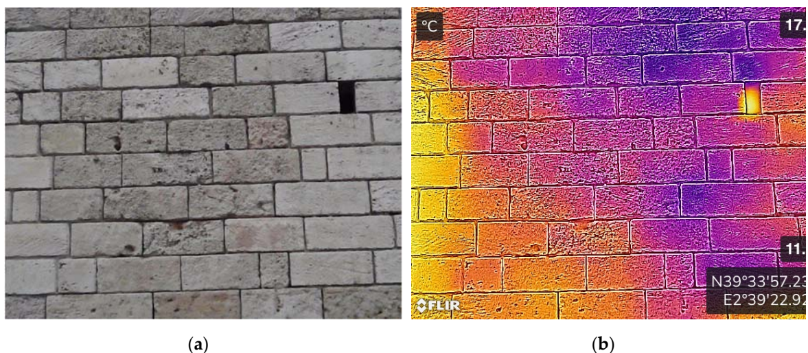
Figure 7. Detail of the southern enclosure wall of the Cathedral of Palma de Mallorca: (a) image captured by a camera, where different ashlar of Marés can be seen; (b) thermogram on the photograph in Figure 7 (a), where the differentiation between the different ashlar is practically non-existent (photographs by the author).
