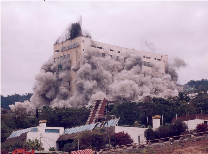
Figure 10. Implosion of Hotel Atlantis [11].
