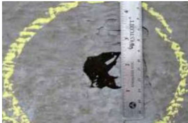
A finish displacement in the top coat of the BUR system
