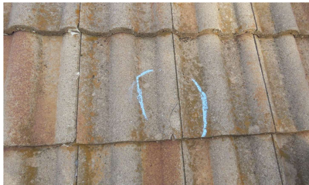
A crescent-shaped crack in concrete field tile with associated spatter mark
