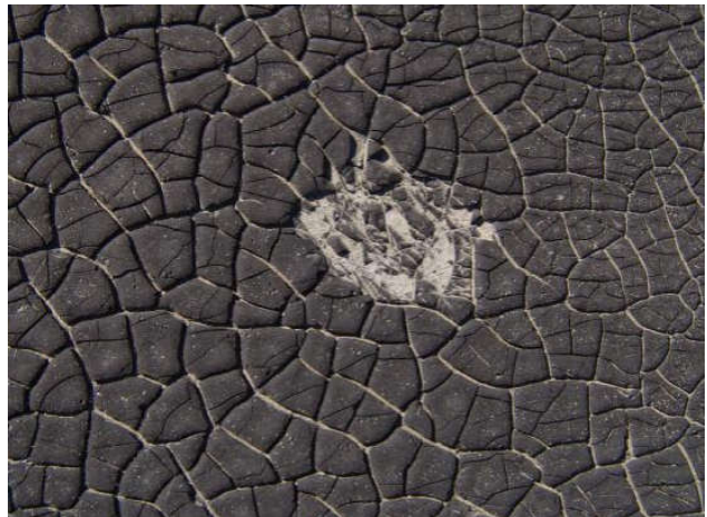
Circular cracks in BUR membrane with associated dull interiors exposed
