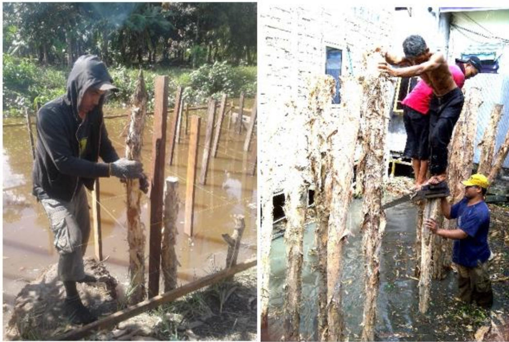
Figure 7. Galam piling with manual method.
