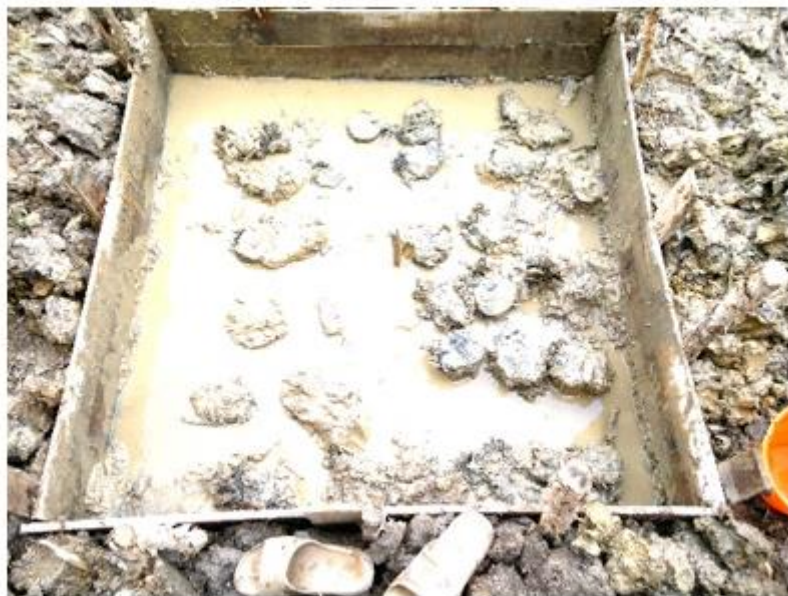
Figure 6. Galam Pile Arrangement for Foundation.
