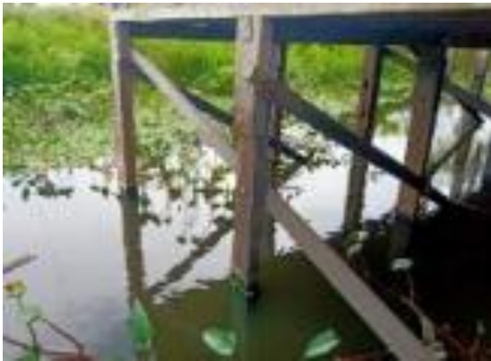
Figure 9. Wooden Pillar Foundation in Swampland.
