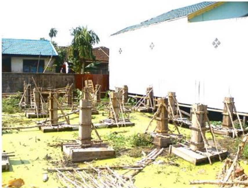
Figure 3. Concrete foundation in swampland.
