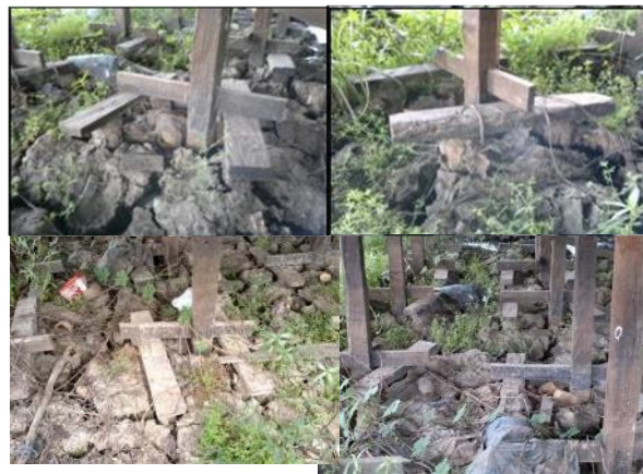
Figure 3. 'Sunduk' Arrangement Due to Construction Errors.
