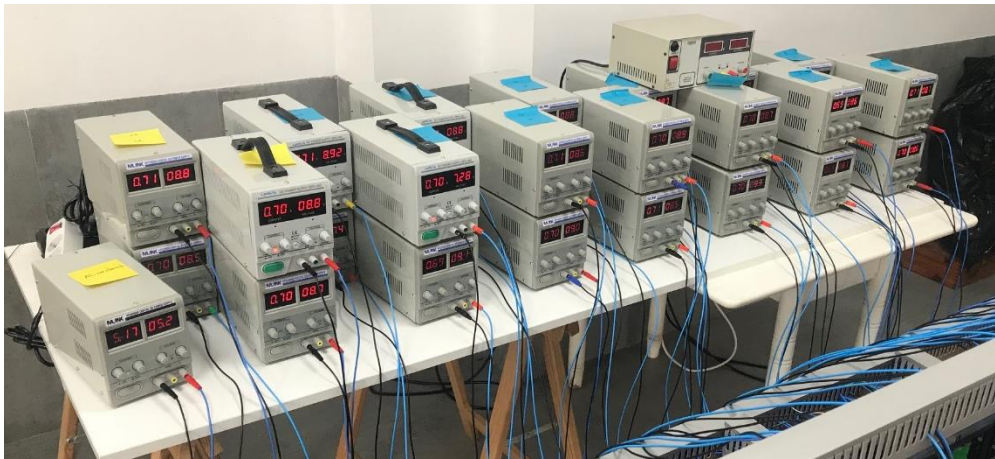
Figure 5. Power supplies for the cells and additional power supply for the process.
