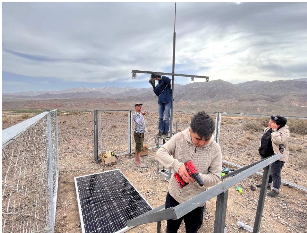
Figure 9. Installation at Boom Gorge.
