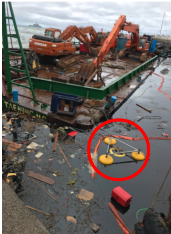
Figure 4. Standard Skimmer working (red circle)
