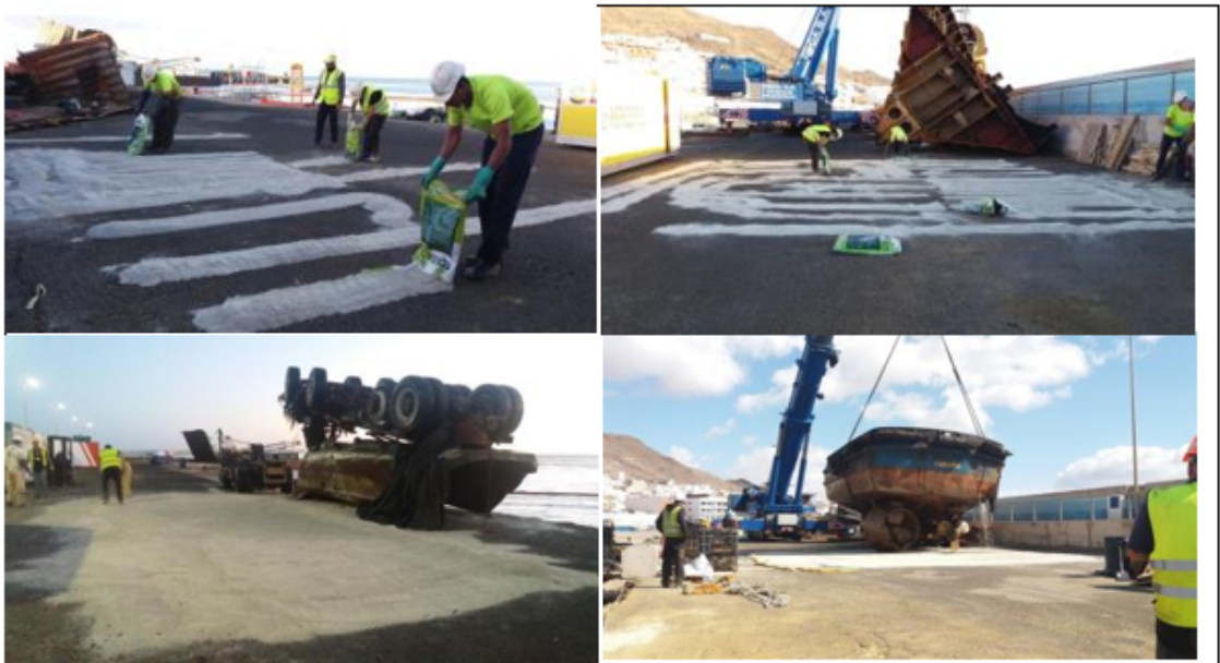
Figura 8. Sequence for the preparation of a bed of oleophilic and highly water-repellent absorbent granules to protect the port soil and prevent water contamination.
