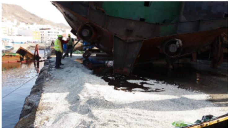
Figure 9. Significant fuel oil spill near the edge of the dock, retained with the combination of granulates and sponges.
