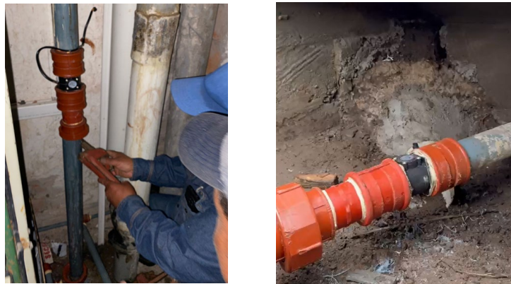
Figure 3. IoT flowmeter in Block B and control center.
