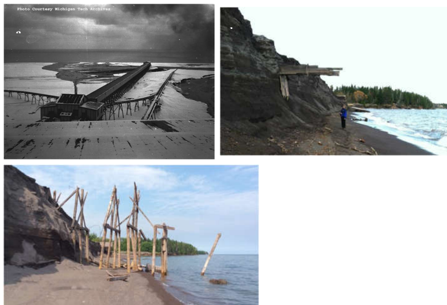
Figure 2. Photos of the Gay Stamp Sand Pile. A) primary wooden discharge launder distributing tailings onto the Gay Pile, around 1922, with smaller sluices conveying stamp sand and slime clays laterally (courtesy MTU Archives). B) Photo of 6-8m high stamp sand bluffs on July 2008, showing a buried small lateral sluiceway protruding out of the pile along the shoreline. Lake Superior waters are to the right; the dark beach sands are stamp sands with slime clay layers. C) Bluff photo from about the same location in 2020, when shoreline erosion (ca. 7-8m/year) reached the buried primary launder wooden support beams, just before bluff removal. Concrete water launder is in background (B & C photos, courtesy W.C. Kerfoot).
