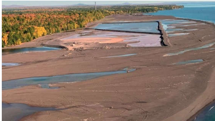
Figure 12. Drone photo of “Berm Complex” (2021), in the stamp sand Pond Field southwest of Gay (stack site). Berm walls were constructed from stamp sand. Plastic pipes pumped dredged stamp sands from the Traverse River Harbor and “Trough” 3-7 km to the Berm Complex. The darker reddish brown sediments are stamp sands between ponds, whereas the lighter pink and orange sediments within the berm walls are recently placed dredged spoils (2020-2021). Notice water percolating through berm walls into surrounding outside ponds. The outer shoreline thickening is also part of construction, intended to protect the Berm Complex from enhanced shoreline erosion. (photo by MDNR).
