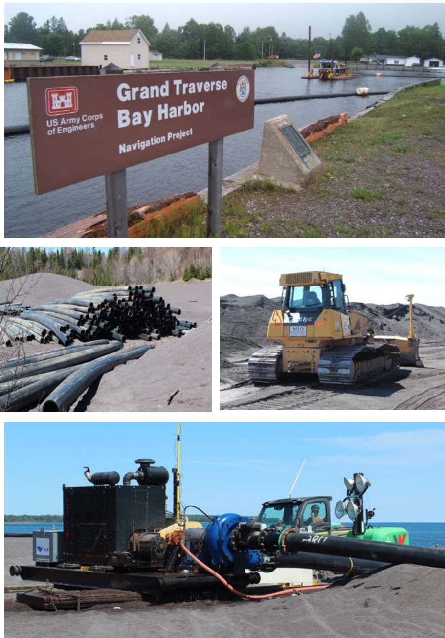
Fig. 11. b) initial dredging begins at the Traverse River Harbor (fall of 2017); c) 5-7 km of pipes and pumping stations used to transport stamp sand from the Traverse Harbor and “Trough” to the “Berm Complex” (2019-2021). (map courtesy of Army Corps, Detroit; photos courtesy W.C. Kerfoot).
