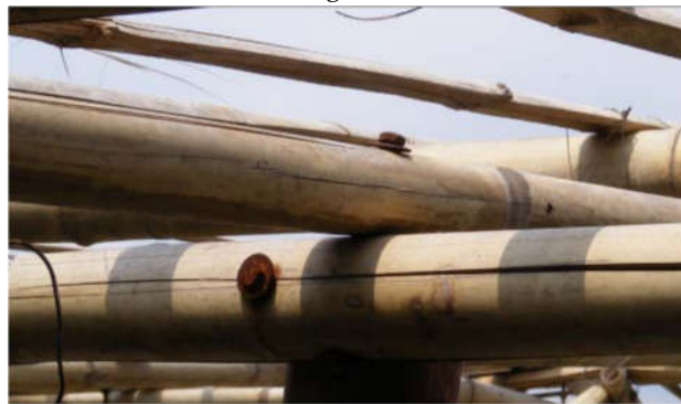
Figure 1 Splitting failure due to bolted connections [14].
