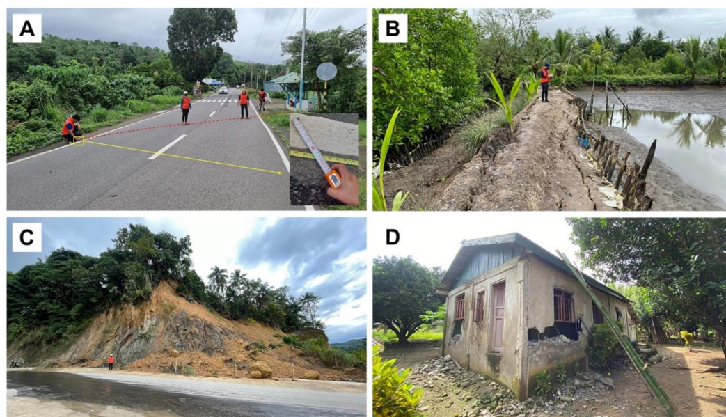
Figure 4. Geologic and structural impacts of the 2023 M_w 4.7 Leyte, Leyte Earthquake. (A) Observed road cracks (red line) along the national highway in Brgy. Poblacion, Leyte coinciding along the trace of the Philippine Fault – Leyte segment [11]. Inset: 2 cm left-lateral displacement measured along the offset road paint. (B) Lateral spreads (cracks) formed on the earth dikes beside fishponds in Palaypay District, Brgy. Poblacion, Leyte. (C) A shallow landslide consisting of soil rock and debris partly covered a road in Brgy. Calaguise, Leyte. (D) Damaged house (concrete hollow block) in Brgy. Belen, Leyte. Refer to Figure 2B for the location of photos.
