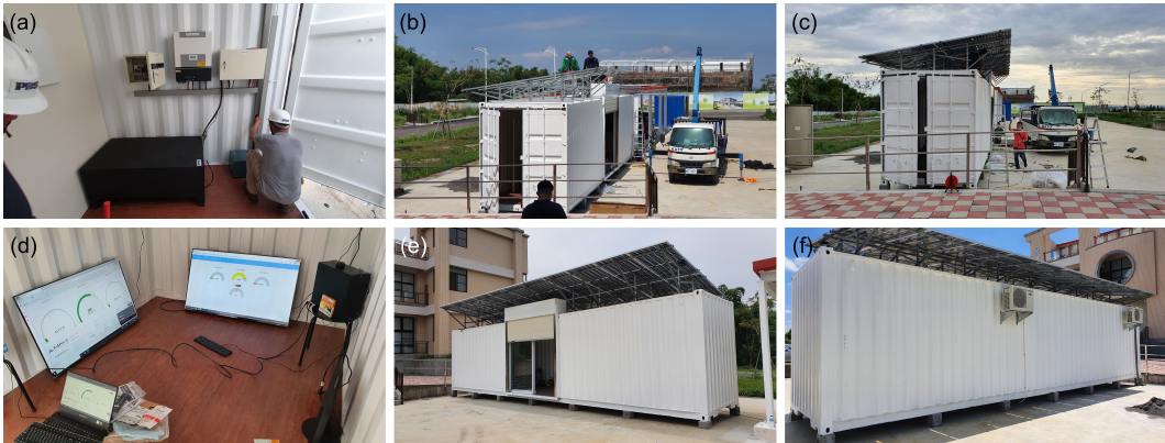
Figure 4. Brief Construction Procedure (a) Installation of the Li-ion battery ESS, inverter, DC and AC distribution, power lines, signal lines, and EMS. (Photo taken on May 9th, 2022) (b) and (c) Erecting the PV panels. (Photo taken on May 10th, 2022) (d) EMS testing. (Photo taken on May 17th, 2022) (e) Installation of electric doors and iron rolling doors. (Photo taken on May 19th, 2022) (f) Installation of air conditioning. (Photo taken on Jun. 2nd, 2022)
