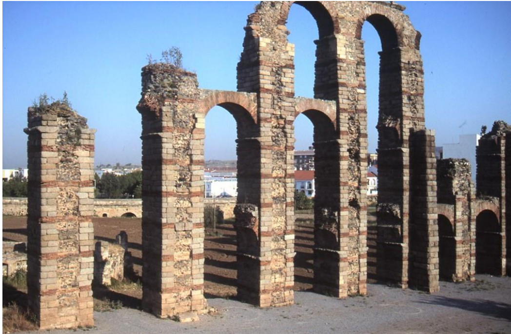
Figure 12. The elevated aqueduct of los Milagros in Mérida, Extremadura. Note the buttress on the fifth pier from the left, and the exposed cores of the first four piers where the buttresses no longer stand.
