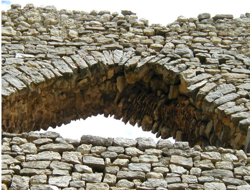
Figure 25. A close-up view of one arch on the elevated aqueduct at Morella showing poorly placed voussoir due to not using centering during construction.
