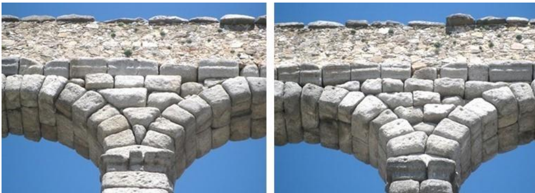
Figure 2. A view of two adjacent spandrels on the aqueduct bridge in Segovia. Note the unique shape of each rock.
