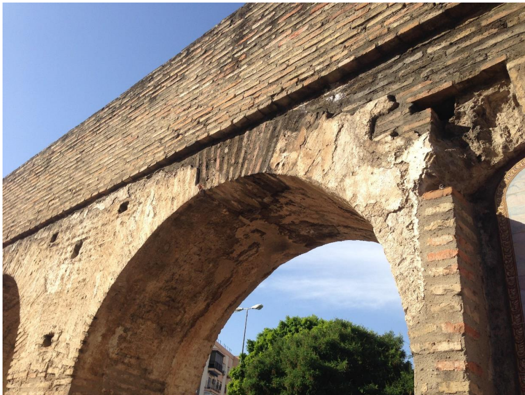
Figure 9. A close-up view of bricks and plaster that characterize the elevated aqueduct in Sevilla.
