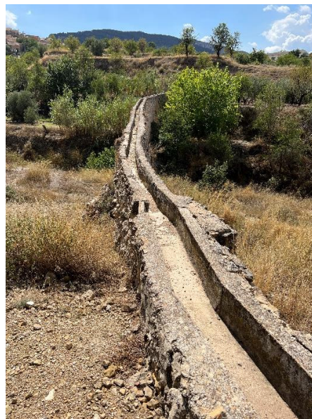
Figure 27. A view along the top of the aqueduct bridge at Biar. Note the narrowness of the aqueduct bridge, its waviness, and buttresses.
