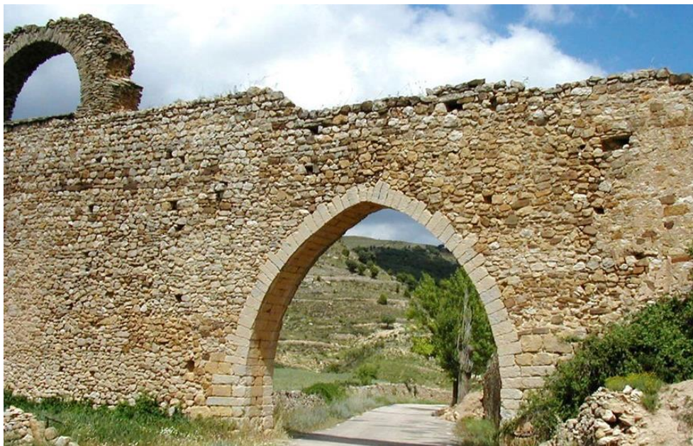
Figure 22. A section of the elevated aqueduct at Morella that is wall-like with a large Gothic arch. Note the large section of exposed core on the right.
