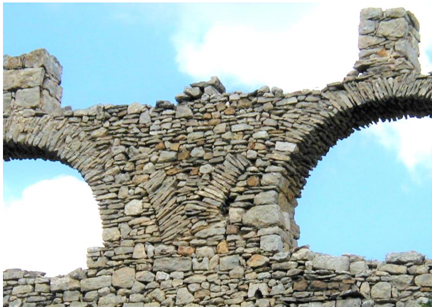
Figure 24. A close-up view of one spandrel of the Morella aqueduct bridge showing reconstruction of two arches.
