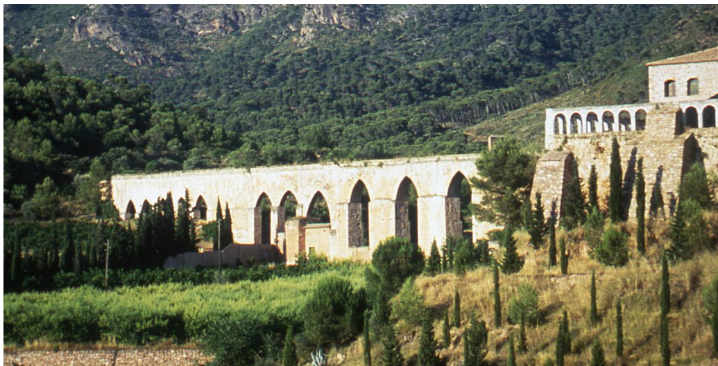
Figure 18. The elevated aqueduct at Puerta Coeli. Note the various thicknesses of piers and the variable heights of the arches. Image by the late Karl W. Butzer, used with permission of his wife.
