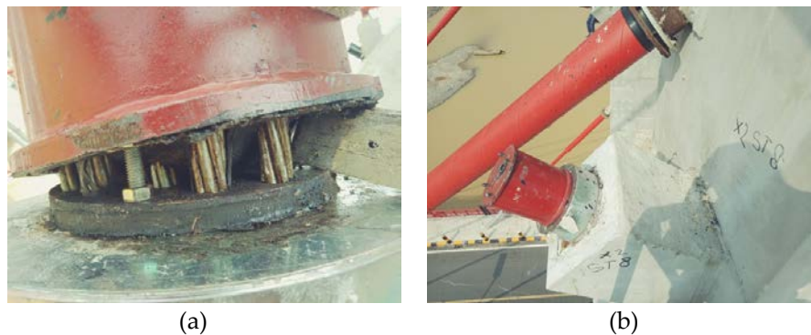
Figure 21. Condition of end anchor on pylon that has been wrapped.
