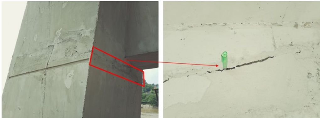
Figure 5. Part of the pylon with unfilled concrete.
