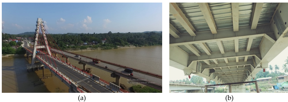
Figure 2. (a) Aerial photo of Sei Dareh Cable-Stayed Bridge; (b) Structural Deck of the Bridge.
