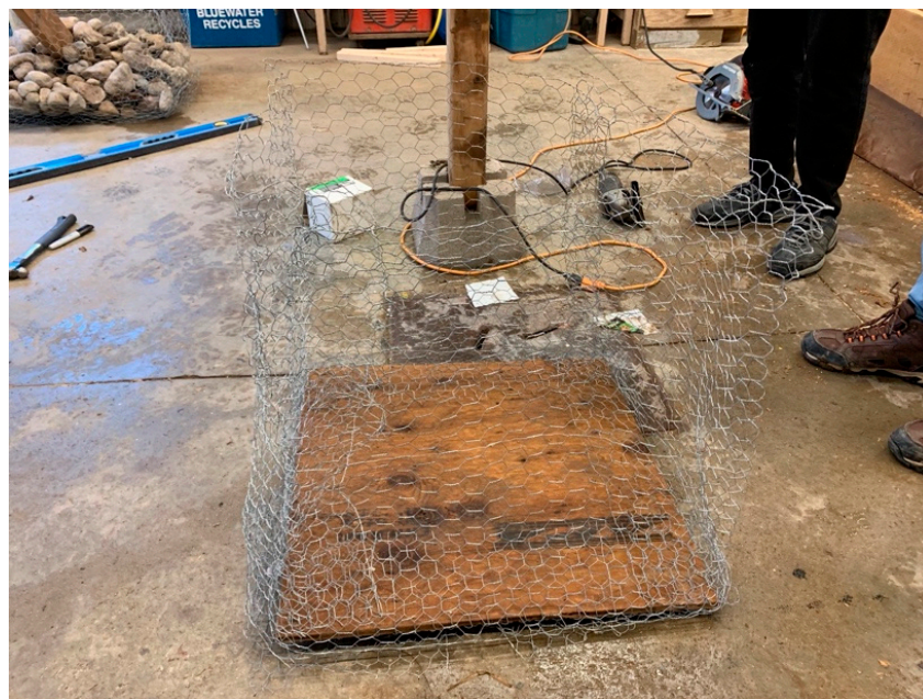
Figure 9. Rock basket formed using plywood and chicken wire.
