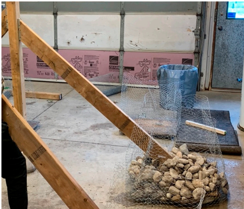
Figure 11. Completed ballast foundation.
