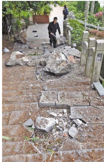
Figure 2. Rockfall in Guilin Diecai Mountain.
