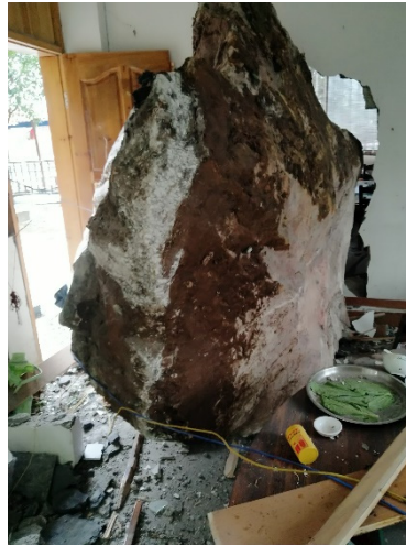
Figure 1. Rockfall into a residential building.
