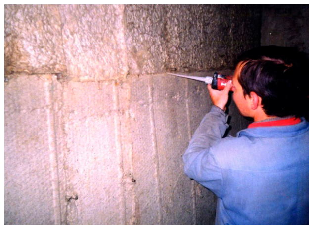
Figure 15. Sealing holes in the heat insulating layer using an injection pistol.
