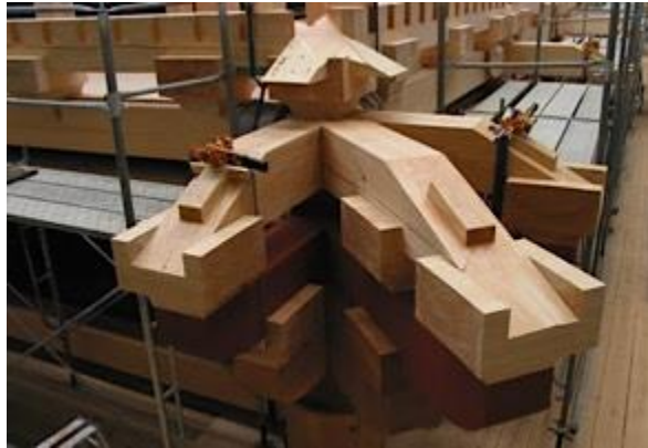
Figure 24. The replacement timbers are assembled as their work position by using traditional techniques (Nara 2006).
