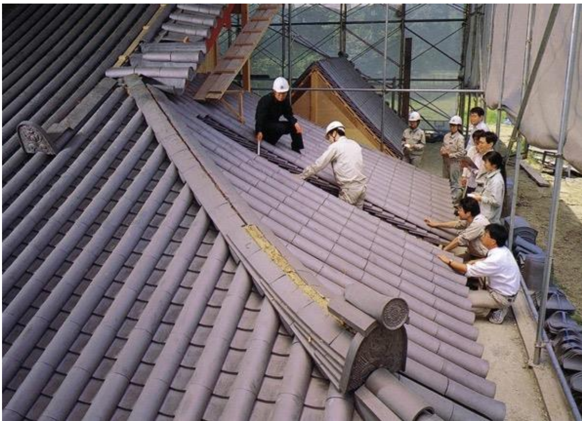
Figure 25. Using authentic material of roof tiles for re-roofing of heritage building (Nara 2006).
