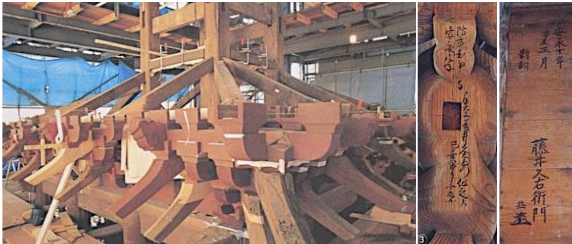
Figure 31. Replacement of decayed timbers with a new one at its primary position and with its original function, conserving the original components by traditional jointing techniques and saving the historical information written by ink (Narra 2004).
