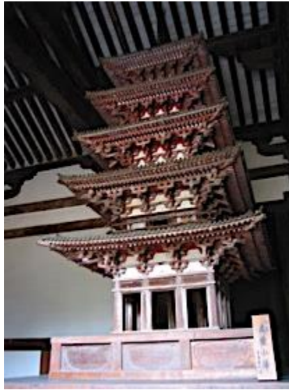
Figure 26. The remaining original 1/5 scale design model of Kairyuuji pagoda, Japan.
