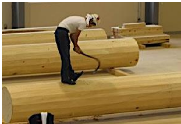
Figure 23. Using authentic material (Hinoki wood) and traditional carpentry tools to represent the historical aspect of replacement timbers (Nara 2006).
