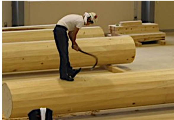
Figure 23. Using authentic material (Hinoki wood) and traditional carpentry tools to represent the historical aspect of replacement timbers (Nara 2006).
