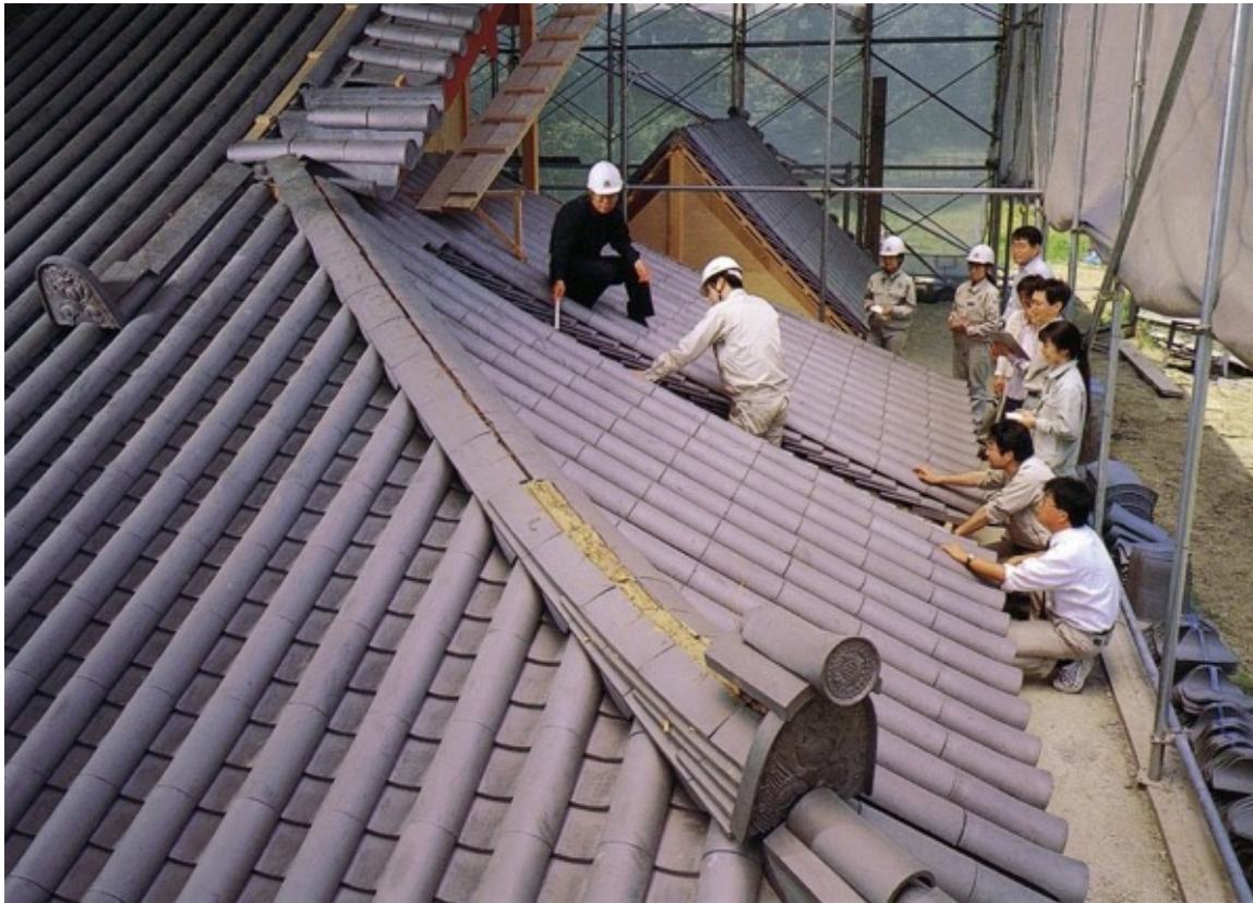
Figure 25. Using authentic material of roof tiles for re-roofing of heritage buildings (Nara 2006).
