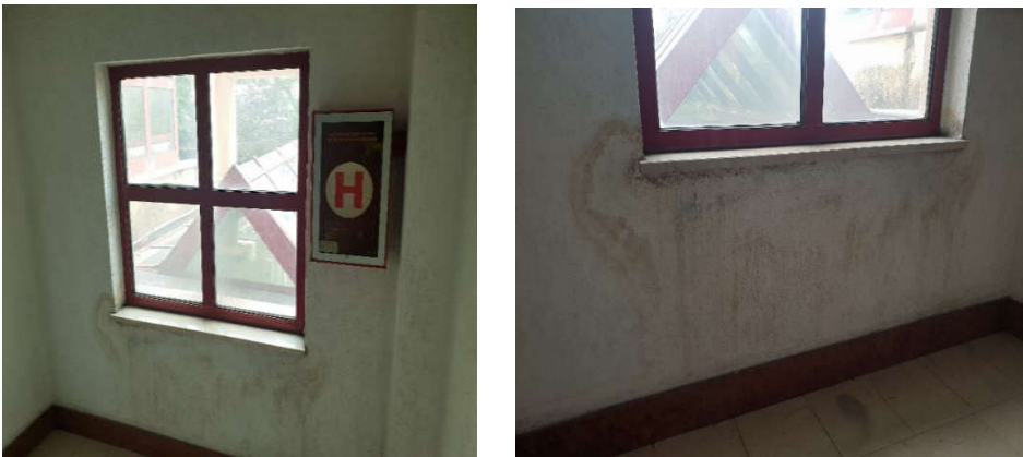
Figures 6,7. The moisture percentage inquiry for a parapet wall, above the ground floor in a masonry building
