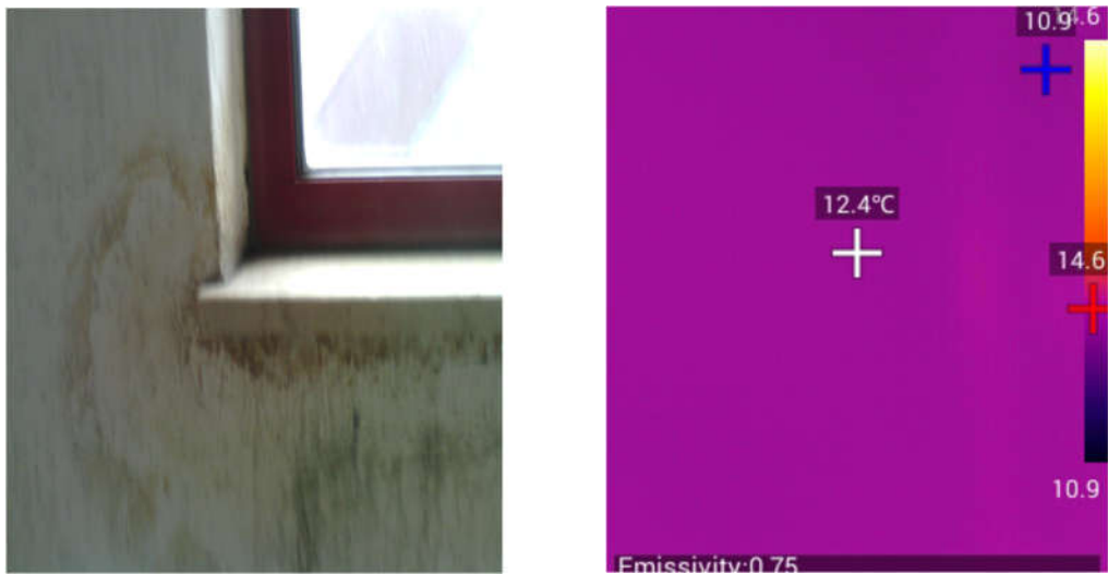
Figure 8,9. A closer photo of a moisture stroken area at a parapet wall above the ground floor and its thermographic snapshot.
