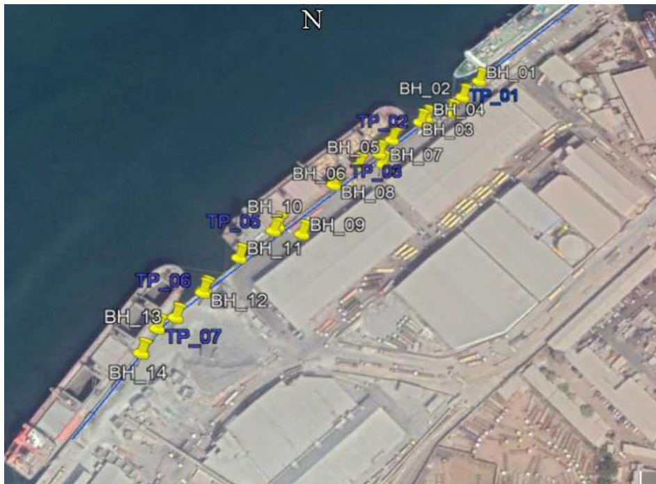
(a) Boreholes location (first study)
