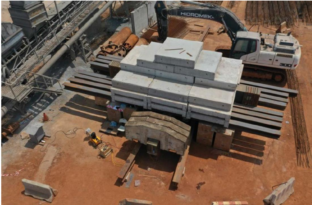
Figure 13. Pile load test set-up.
