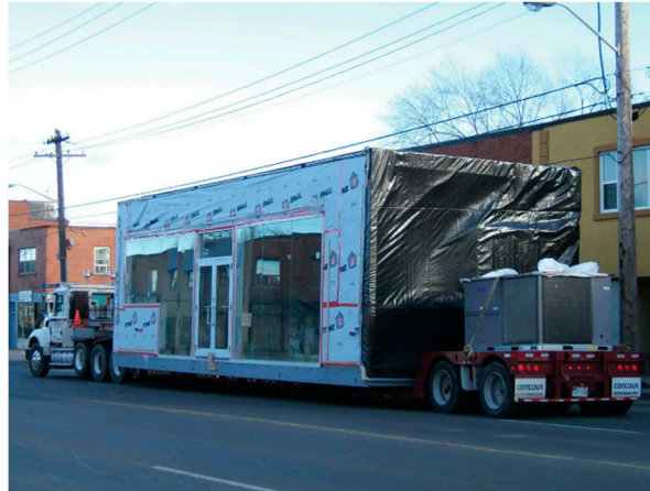
Figure 2. Fully fabricated modular unit with partial finishing transported to the site adapted from [11].
