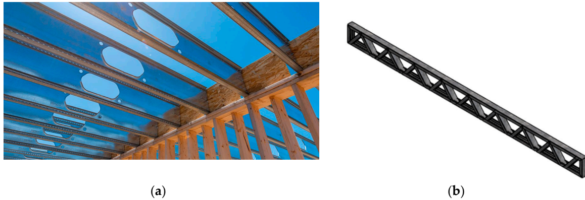
Figure 4. (a) CFS lipped C joists [31]; (b) MVIVO lipped C truss.
