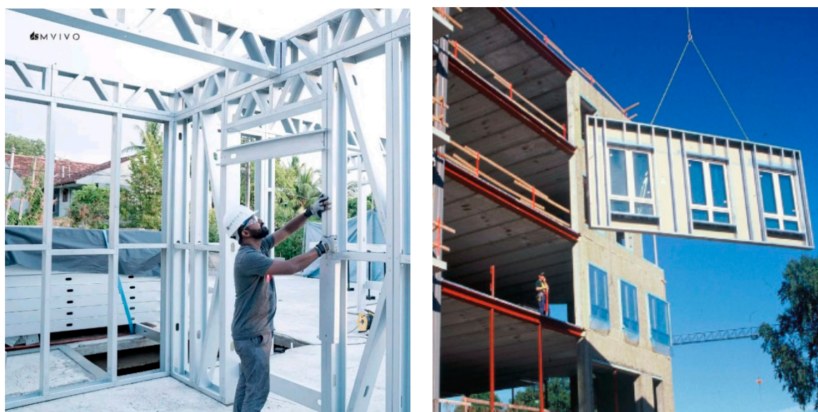
Figure 1. (a) Stick-built construction adopted by MVIVO; (b) Prefabricated curtain wall installed adapted from [10].
