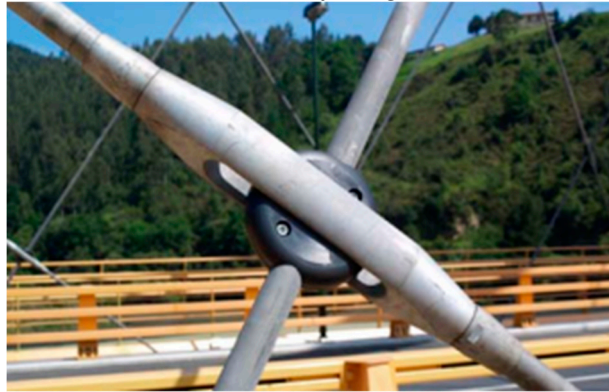
Figure 14. Hanger crossing device in the form of a needle eye [28].
