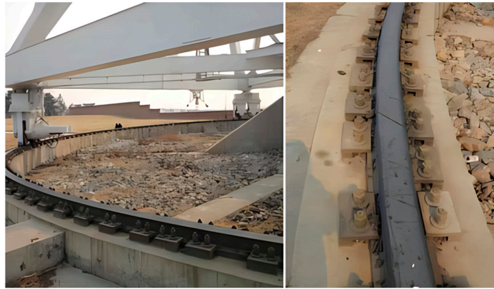
Figure 4. Azimuthal track for large wheel-rail antennas.
