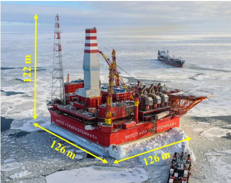
Figure 6. The appearance and basic geometric characteristics of the “Prirazlomnaya” platform [29].
